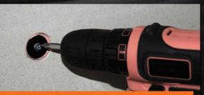
Drill a hole directly through the DClox fastening element and insert the dowel and the screw. Fasten the screw and adjust the panel at the desired distance from the existing wall.
